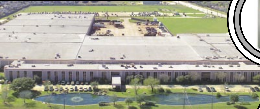
North America Headquarters & Manufacturing Facilities (Houston, TX)
